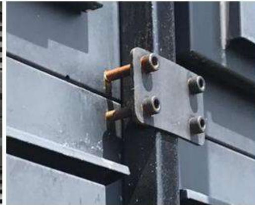
Traditional Iron cabinet only has metal plates for fixed cabinets together, more difficult to make cabinets to be alignment with each other
